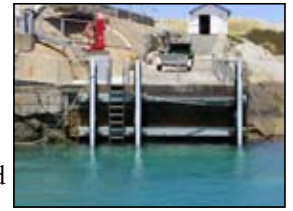
The Refurbished Jetty P. Bourke
