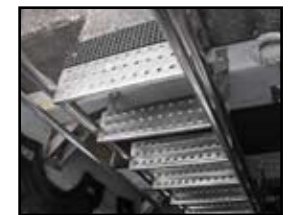
Close up of new ladder & beams. MW
