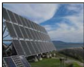
New panels up on the frame, old panels below. - MW
