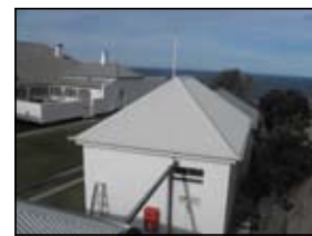
Oil Shed with new roof. MW
